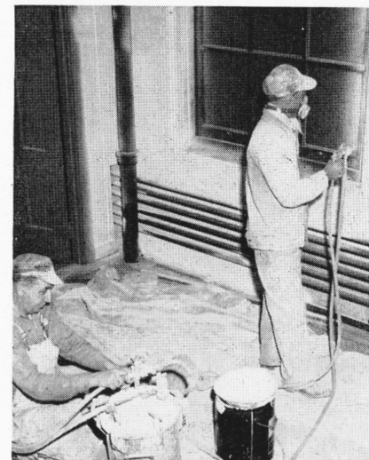
Andrew Pentino and John McAuliff, Scovill painters, sprayed paint on the walls of Seventy-one Building, recently. Andy was handling the spray gun on this occasion.
